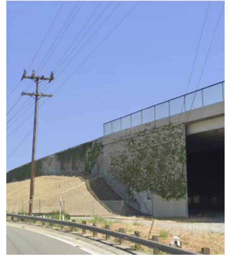
After Removal of Pylon Sign
