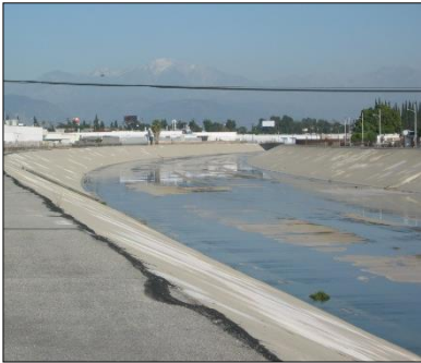
Flood Control Channels
