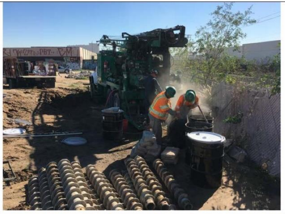
Photo 4. View of cement mixing.
