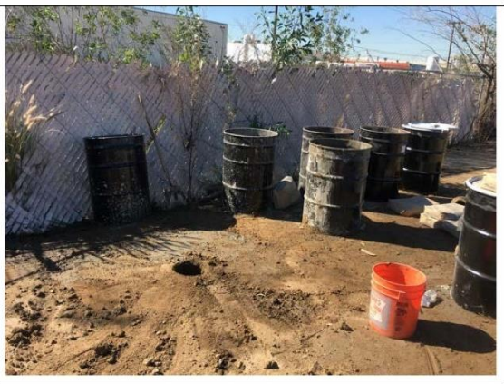
Photo 6. View of well with cement settling and waste soil drums.
