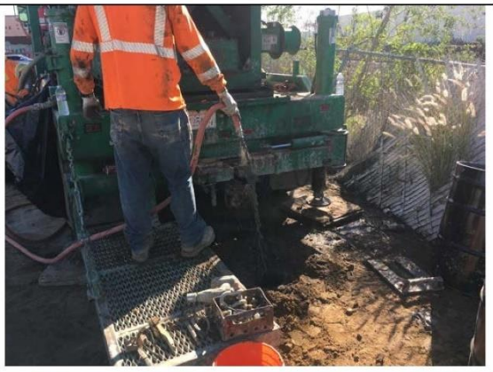
Photo 5. View of cement being poured into the well.
